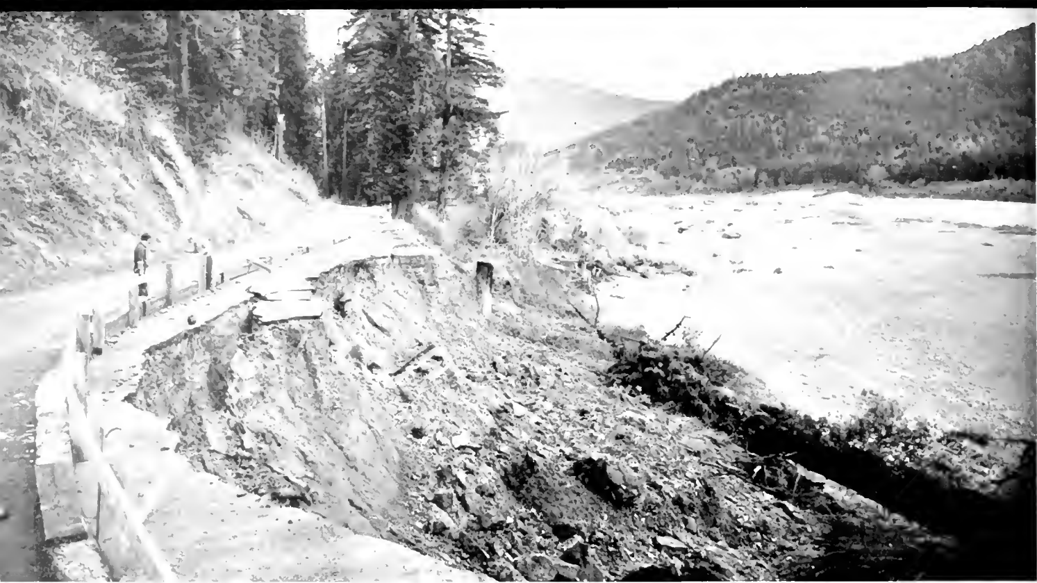
Redwood Highway on Eel River in Humboldt County damaged by flood waters where timber deflectors have been placed to protect bank
